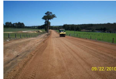
(Perup Road construction works)
