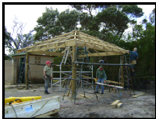
(Pictured above: Construction of fish cleaning facility in Walpole.)
