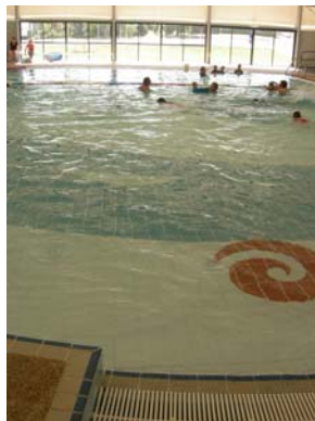
A sloping graded entrance makes access to the Manjimup Swimming Pool easy for all
