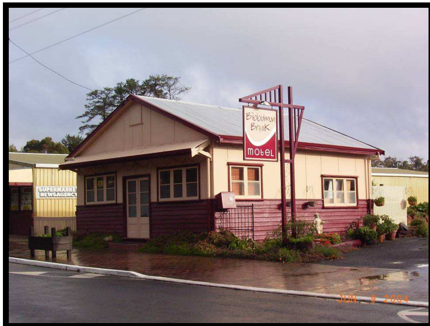
The old R&I Bank in Northcliffe has been converted for accommodation hoping
