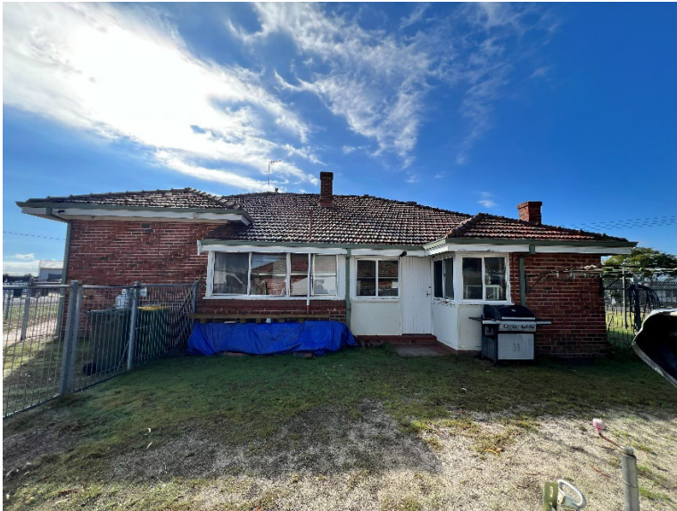
Figure 4 View of southwest elevation.
