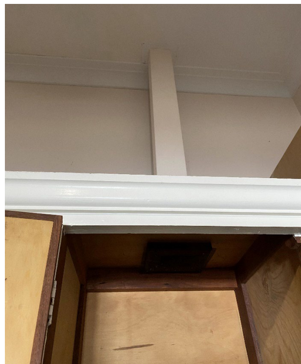
Figure 57 Vent in roof of built in pantry
