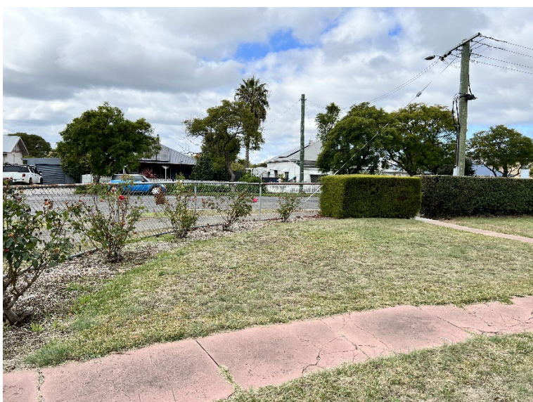
Figure 8 View of the front yard showing the original hedge and rose garden. Cracks on concrete path evident.
