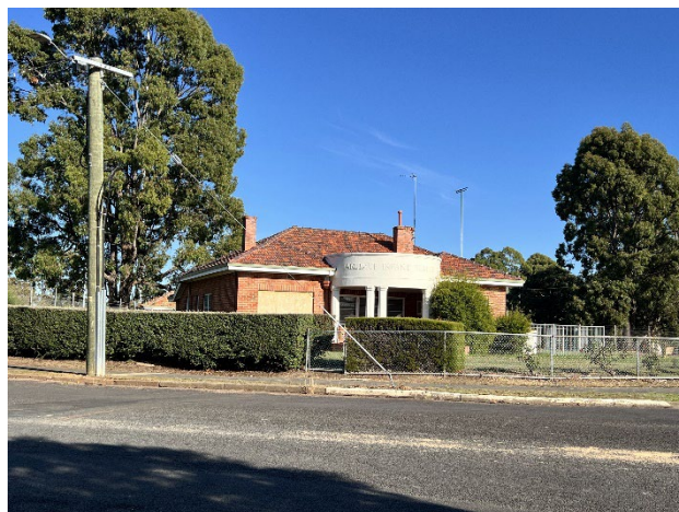
Figure 11 View of east elevation with hedge and mesh fence on the site boundary.
