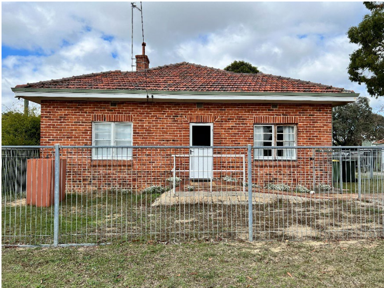
Figure 2 View of northwest elevation with modular panel fencing in the foreground.
