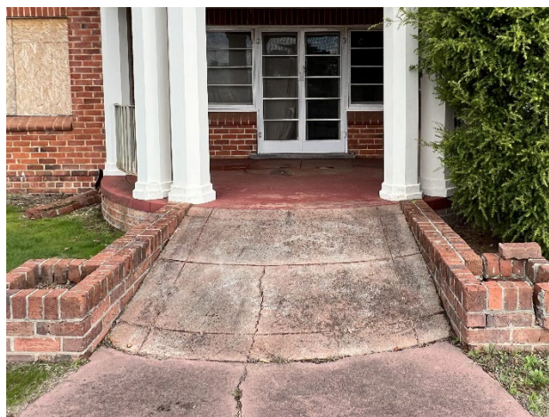
Figure 22 View of concrete entrance ramp.
