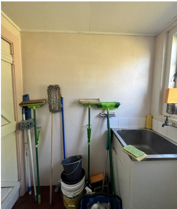
Figure 59 Laundry trough with tiled splashback is intact. Scuff marks and stains to walls, ceiling and trims.
