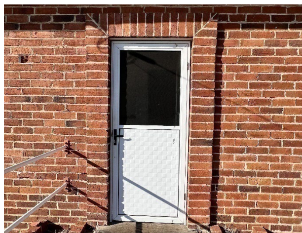
Figure 27 View of brick surround that frames the north-west entrance door.
