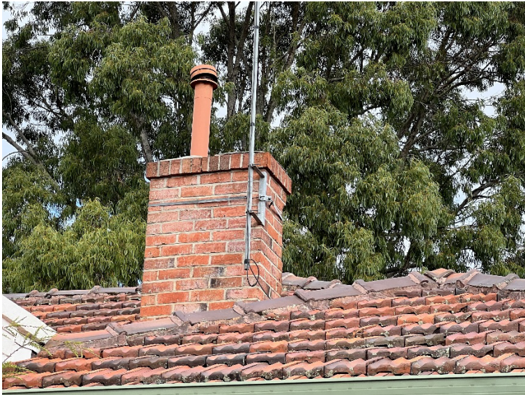
Figure 11 Antenna mast fixed to chimney stack.
