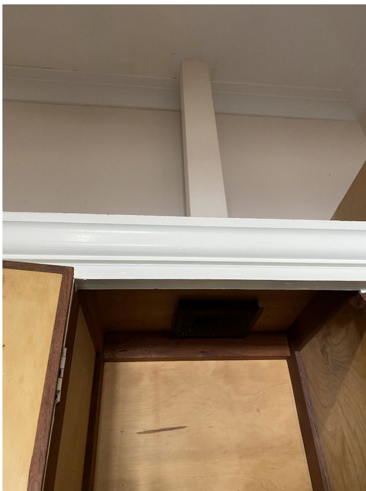
Figure 43 Original pantry cabinet with passive ventilation system (air exhaust).
