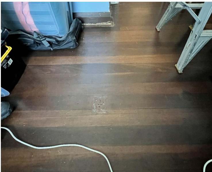
Figure 38 Evidence of central support post location on floorboard.
