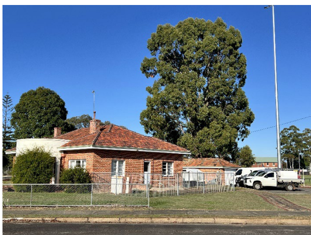
Figure 12 View of northeast corner with steel and mesh fence on the site boundary.
