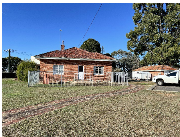
Figure 13 View of north elevation with modular panel fence in front.
