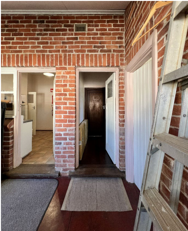
Figure 42 View from enclosed verandah showing corridor to visitor ablutions, kitchen to left
