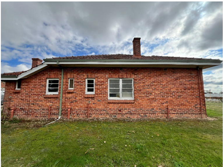
Figure 3 View of southeast elevation
