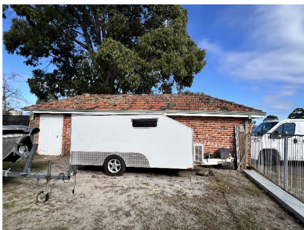
Figure 18 View of rear shed facing west.
