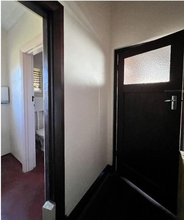
Figure 40 View of the hallway access to washroom and WC 1.
