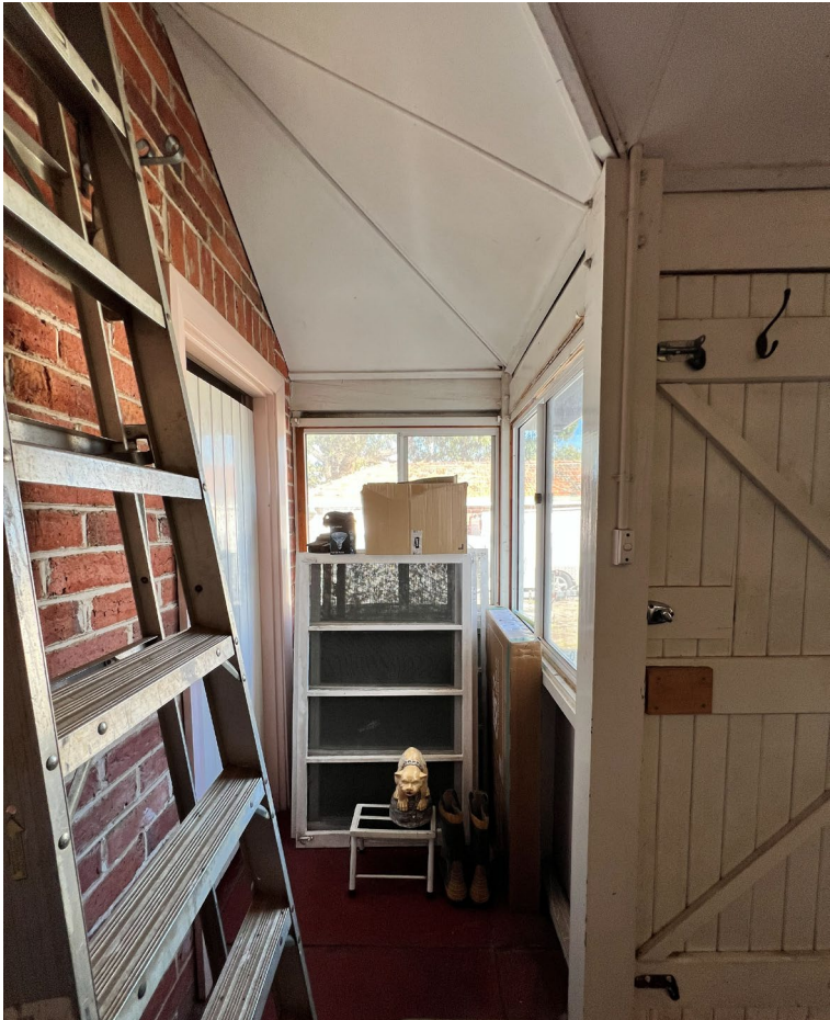
Figure 57 Aluminium framed windows to verandah enclosure.
