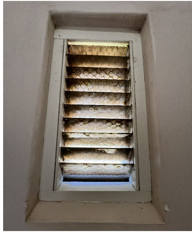
Figure 43 Louvred windows to visitor toilet
