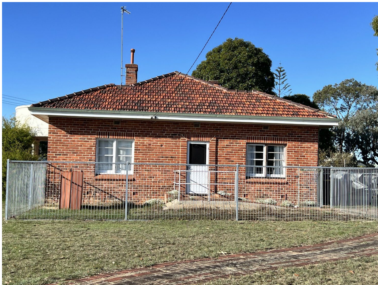
Figure 25 View of northwest elevation with modular panel fencing in the foreground.
