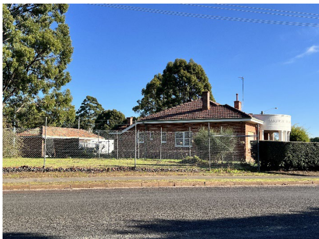
Figure 10 View of south elevation with steel & mesh fence on the site boundary.
