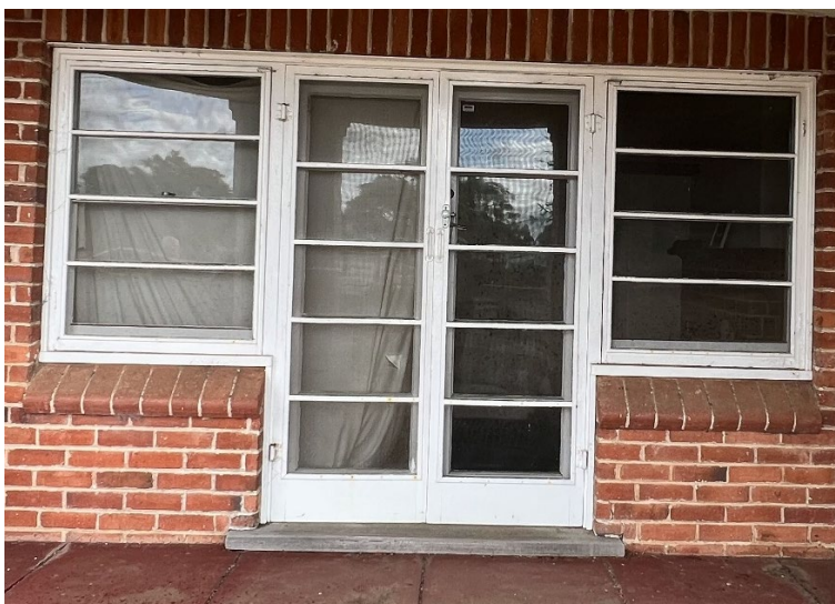
Figure 24 Main entry double door and flyscreen. Double hung sash sidelights with casement flyscreen. Timber door threshold generally aged.
