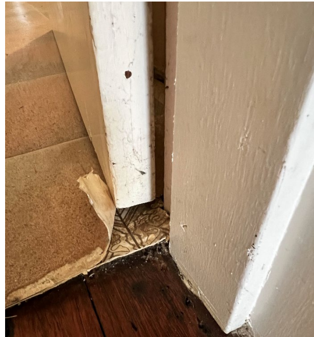
Figure 55 Vinyl layers to kitchen floor
