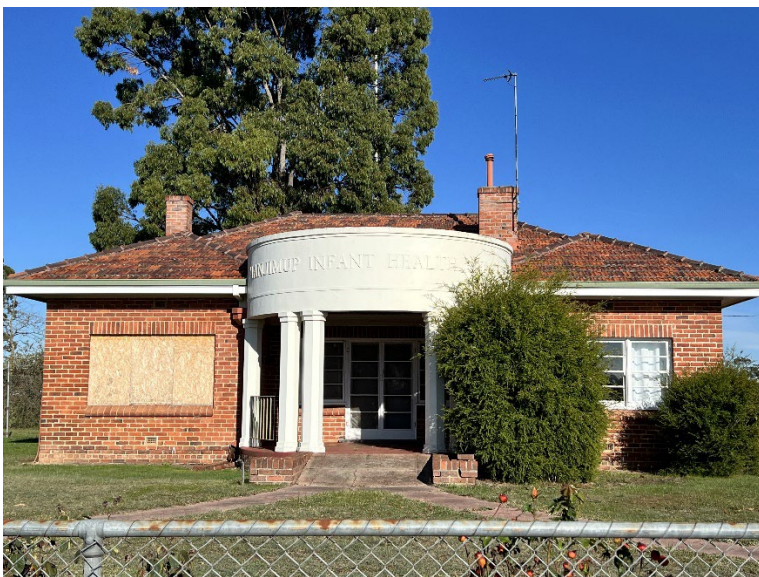
Figure 5 View of northeast elevation. Glazing is missing on the west side window which has then been boarded up.
