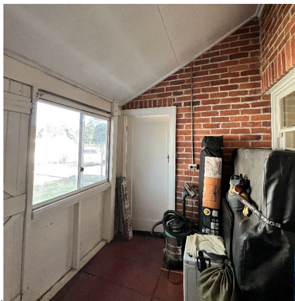
Figure 60 Enclosed verandah looking towards sleep-out door
