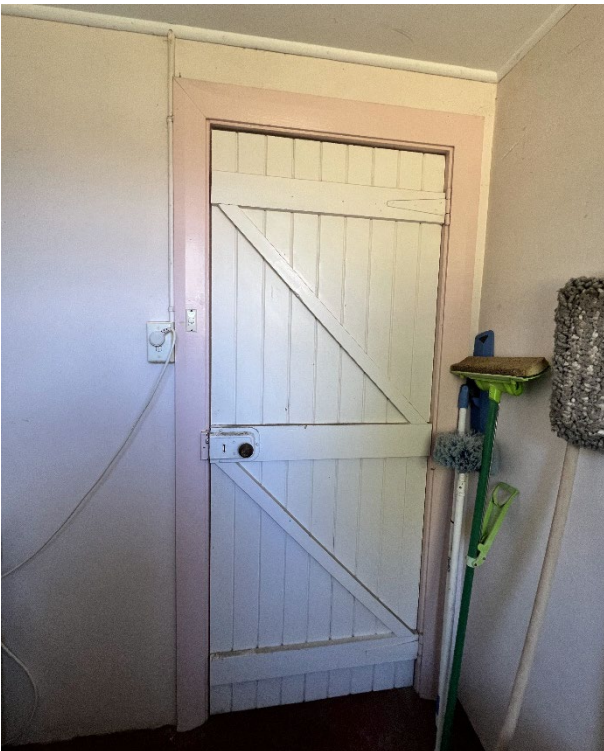
Figure 64 Rear of laundry door
