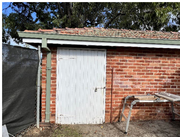
Figure 67 Timber panelled door to east elevation
