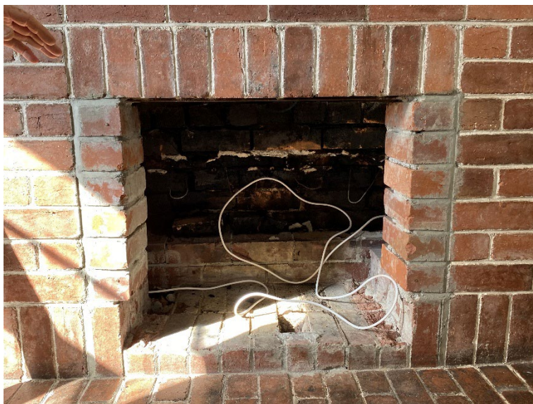
Figure 48 Living room fireplace
