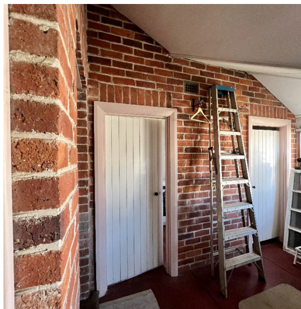
Figure 61 Doors to laundry and nurse toilet off enclosed verandah
