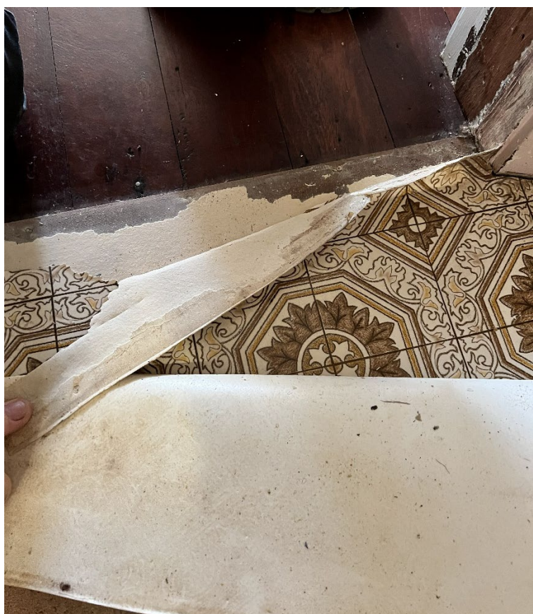
Figure 42 Layers of floor covering to kitchen floor.
