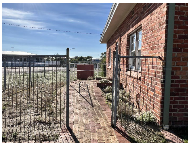
Figure 26 View of ramp to north-west entrance.
