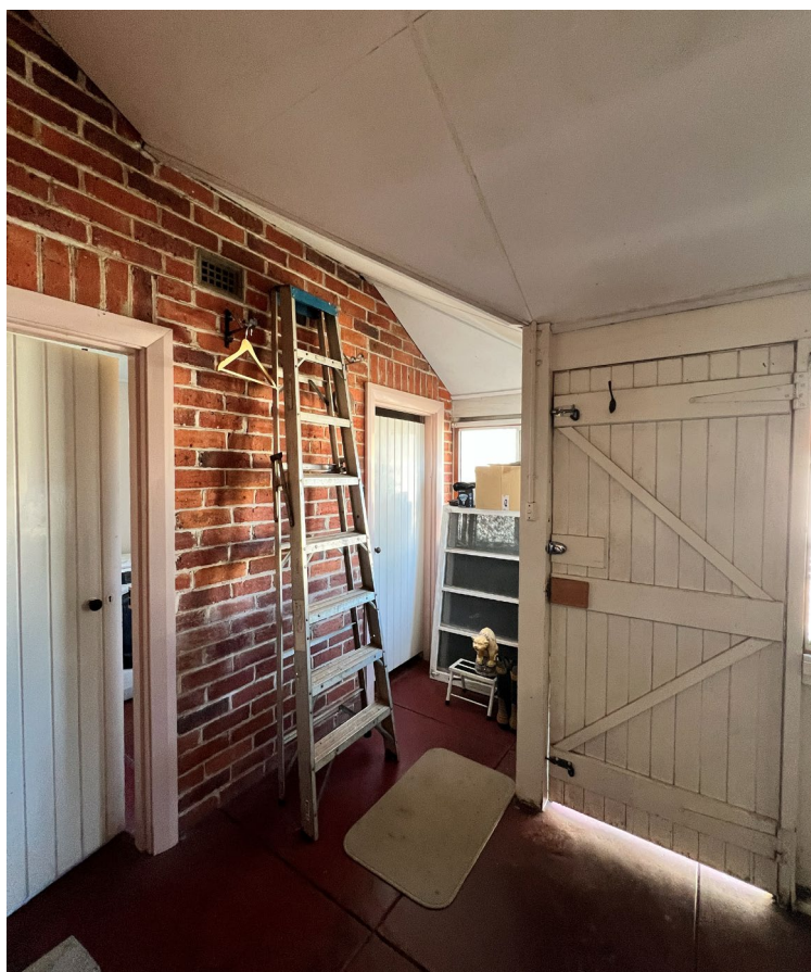
Figure 55 View of verandah with doors to laundry and WC2.
