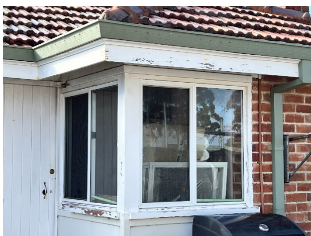
Figure 29 View of the south wing of the western façade.
