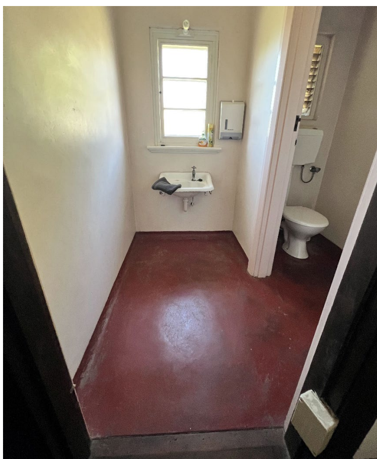
Figure 50 View of washroom with WC 1 to the right.
