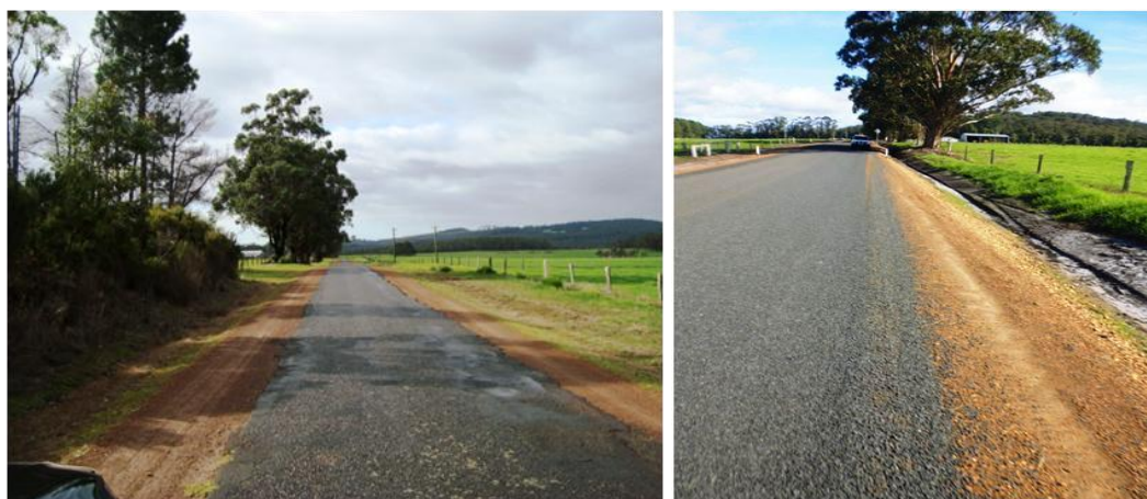
Bridge Road before (Left, looking east) and after (right, looking west) Construction & Sealing
