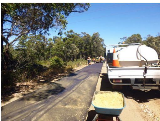
Sealing of Perup Road shared path.
