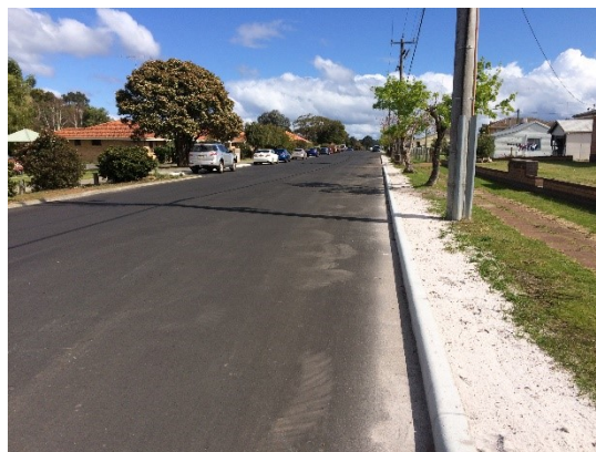
Ipsen Street, Manjimup. New asphalt seal and new kerb line, relocated to provide room for street trees to grow.
