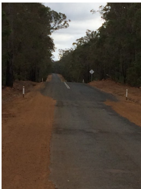
Perup Road showing new construction where it meets the single seal width road it has replaced.
