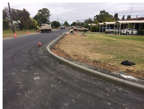
New kerbing placed prior to asphalt re-sealing on Edwards Street, Manjimup
