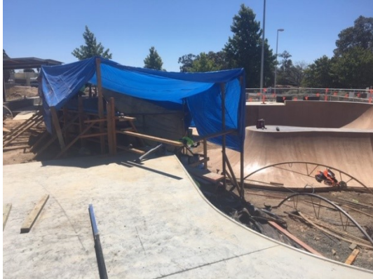
Trying to keep the sun off during a pour on the new skate park
