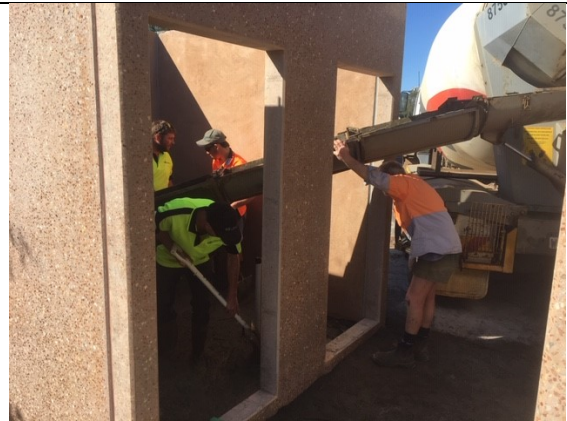
Floor being poured in the New Ablution Giblett Street
