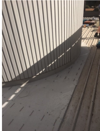
Curved Flashing being installed to prevent roof leaks in refurbished State Timber Museum
