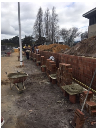
Retaining Wall construction Coronation park
