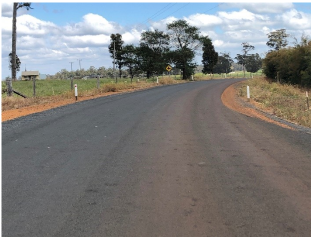
Rip, reform and seal project, Springall Road Manjimup
