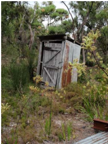
Photo 3: an example of the current effluent disposal systems within Reserve 19787.
