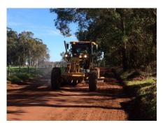
The main purpose of patrol grading is to provide a good running surface and to form crossfalls in the road so that water runs off and does not pool. Water pooling on roads causes pot holes when vehicles drive through them. Moisture is a critical component in patrol (maintenance) grading, which is best done when the gravel has the right amount of moisture in it.
